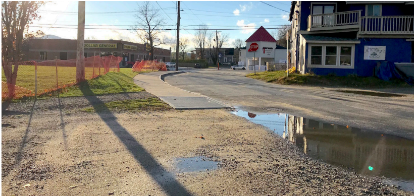
Impervious surface and a poor drainage pattern creates pooling on Mill Street.
