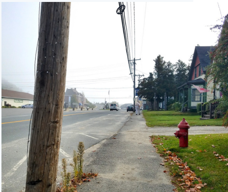
Asphalt sidewalks are level with the roadway. With no striping they look just like the road or shoulder.
