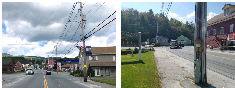
Above ground utilities have a big impact on the streetscape.
